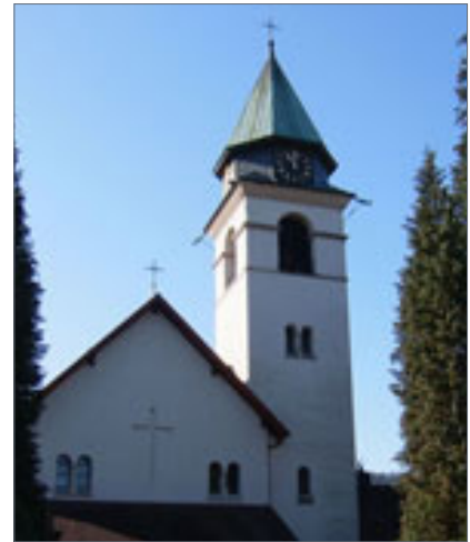
Church with AFILS system installed
